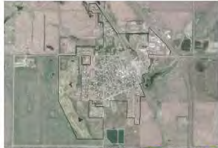
City of Underwood • Fire
